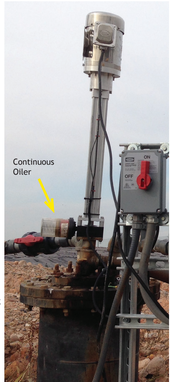
Continuous rod oiler attaches to seal plate
